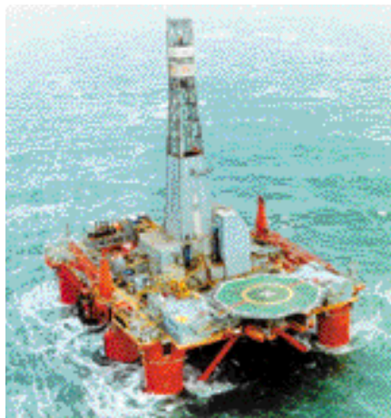
Left: The Transocean Paul B Loyd Junior deepwater semi-submersible drilling rig is capable of working in harsh environments and water depths up to 600 metres. Top right: A basket star clings to a piece of subsea machinery. Bottom right: Subsea 7 work-class Pioneer HD ROV connected to its tether management system for deployment. It is equipped with seven and five function manipulator arms, camera systems on moveable pan and tilt unit and high-power subsea lighting. All these tools make it an ideal vehicle for scientific operations.
